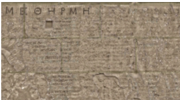
Figure 3. A sample of the plotting of the epigraph. The deterioration of the surface is clearly visible
